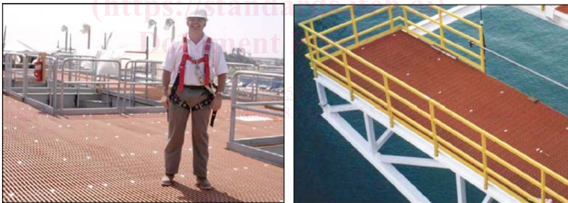
FIG. X1.1 Grating Floor Systems as Used Offshore
