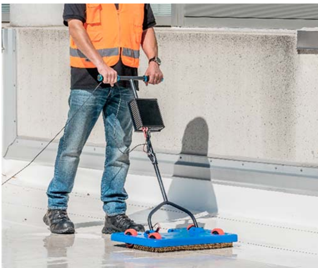
FIG. 2 Testing a Horizontal Membrane with a Scanning Platform
