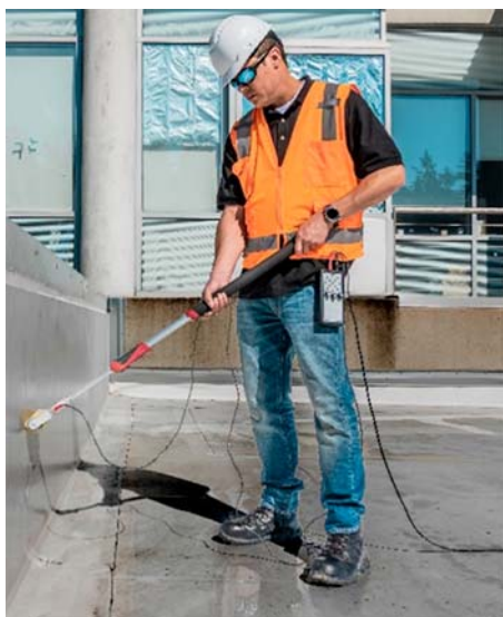
FIG. 4 Testing a Detail Area with the Vertical Surface Unit
