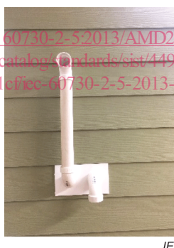
Figure 102 – Typical installation of the independent combustion air supply for room independent operation
