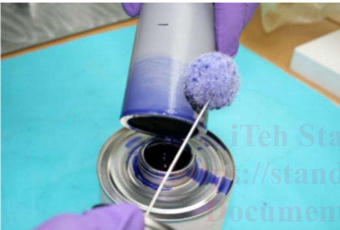
FIG. 12 Apply primer to the pipe end beyond the mark delineating the depth of the fitting socket.
