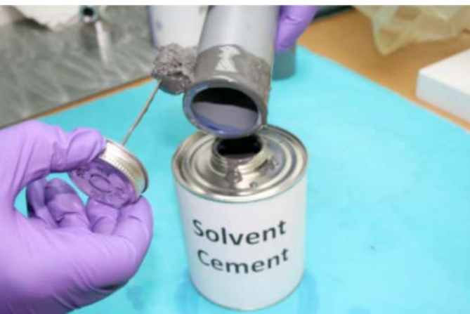
FIG. 13 Apply a full, even layer of solvent cement to the pipe end beyond the mark delineating the depth of the fitting socket.
