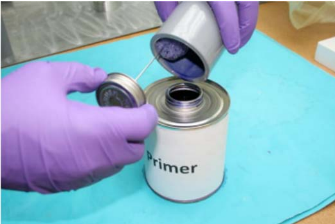
FIG. 11 Apply primer to the fitting socket.
