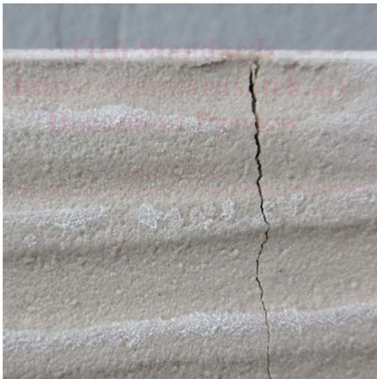
FIG. 8 Crack, Basic
