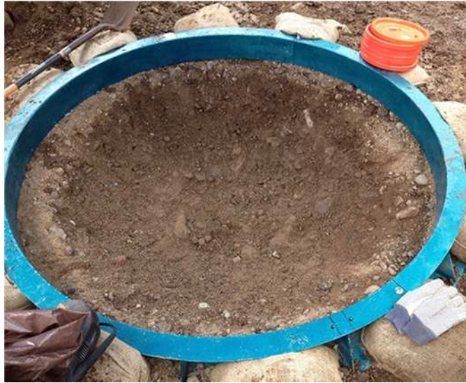
FIG. 4 Test Pit Excavation
