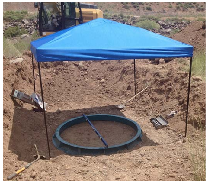
FIG. 1 A 6-ft [1.8-m] Diameter Metal Ring for Determining In-Place Density
