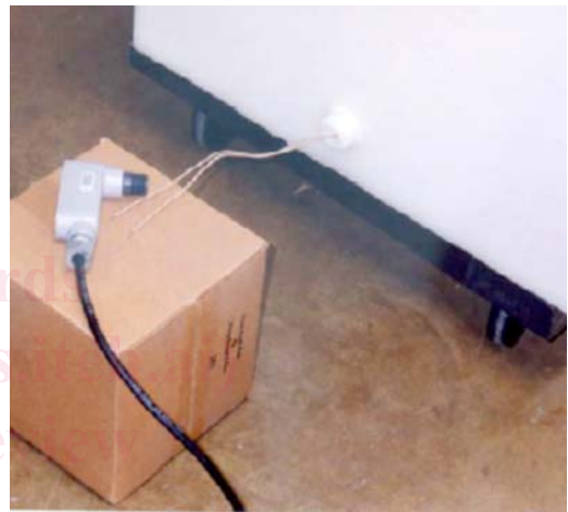
FIG. 7 TC Heater Installed in Tank Exterior
