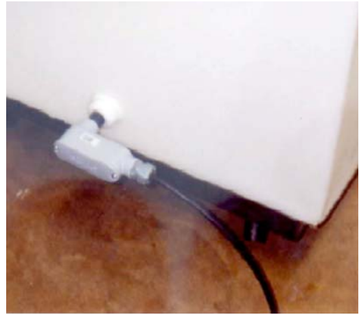
FIG. 6 Heater Conduit Boc Installed on Tank
