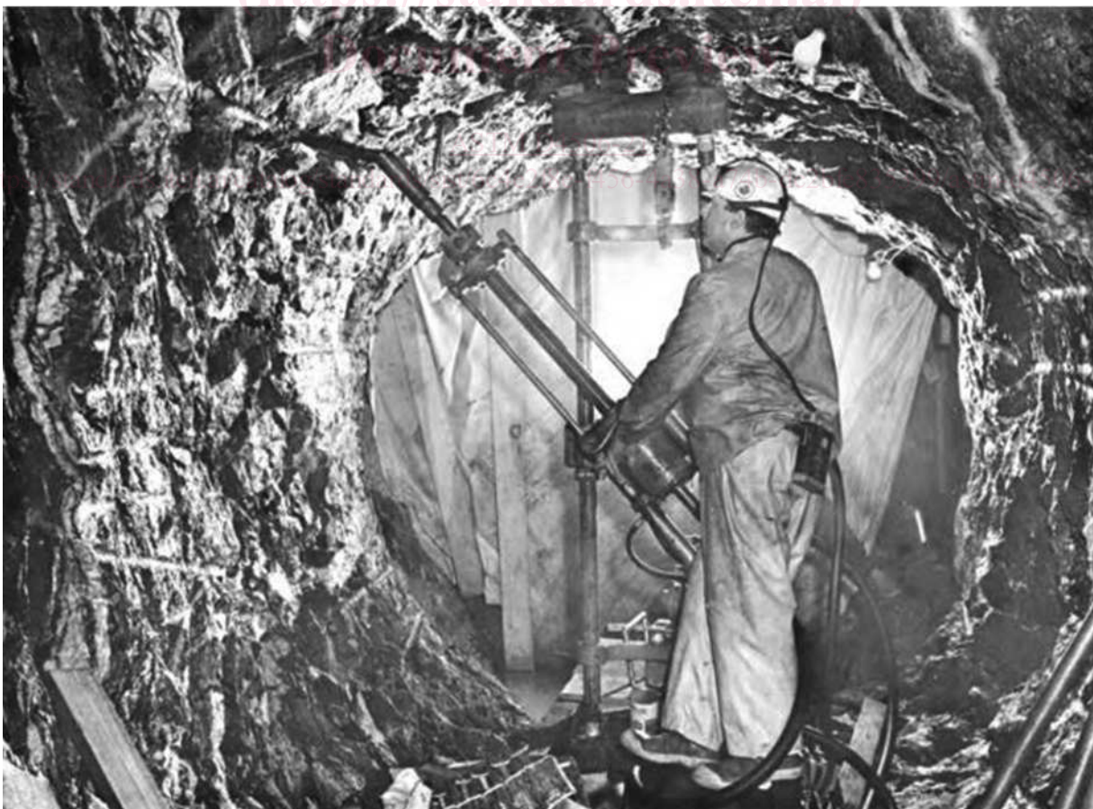
FIG. 5 Drilling Instrumentation Holes for Radial Jacking Test (1) Courtesy of US Bureau of Reclamation
