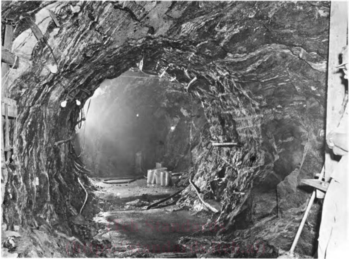
FIG. 4 View of Final Radial Jacking Test Chamber Excavation and After Installation of Extensometers (1) Courtesy of the US Bureau of Reclamation
