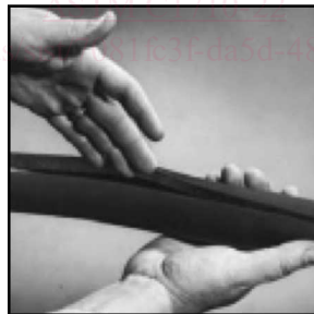
FIG. 3 Apply Unslit Insulation to Straight Pipe
