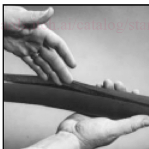
FIG. 3 Apply Unslit Insulation to Straight Pipe
