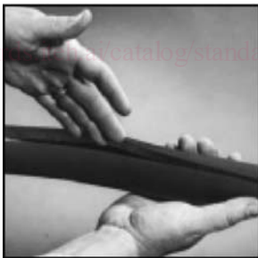
FIG. 3 Apply Unslit Insulation to Straight Pipe
