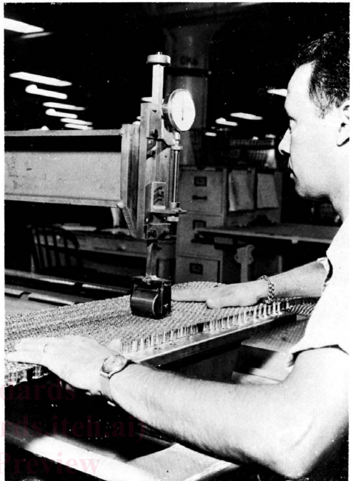
FIG. 1 Roller-Type Thickness Tester
