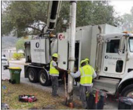
FIG. 3 Vacuum Excavation Equipment
