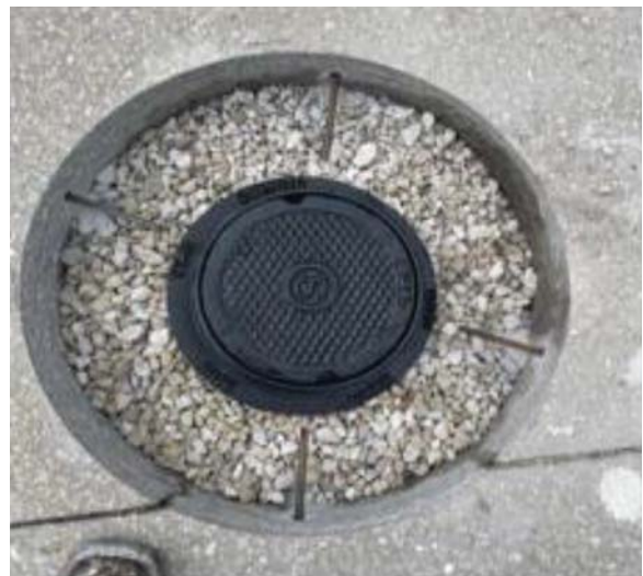
FIG. 5 Cored Pavement with Dowels
