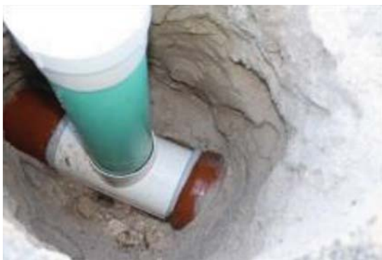
FIG. 4 Vacuum Excavated Borehole
