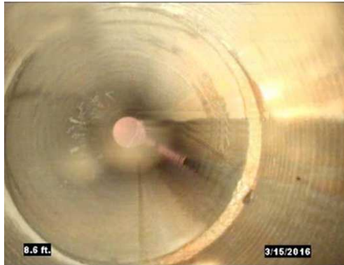
FIG. 13 Joint Offset
