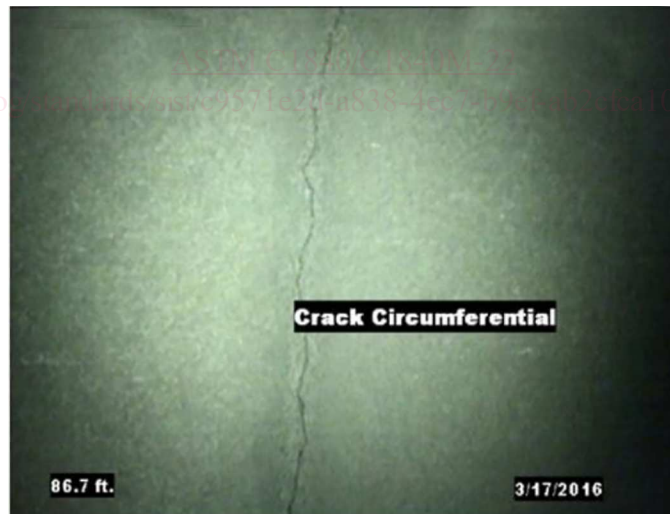
FIG. 6 Circumferential Crack
