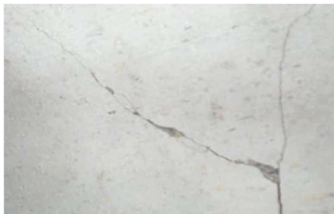
FIG. 9 Multi-Directional Crack
