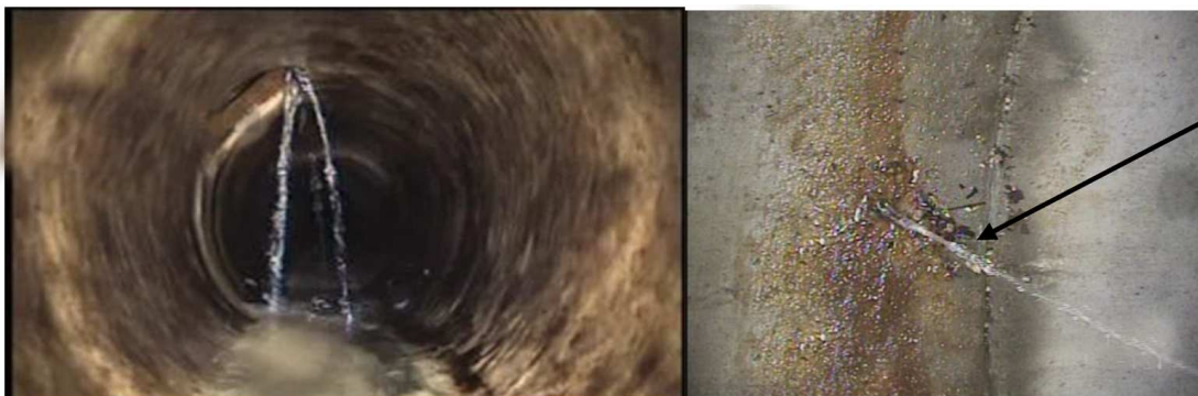
FIG. 12 Level 3 Infiltration
