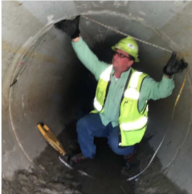
FIG. 1 Person Entry Inspection
