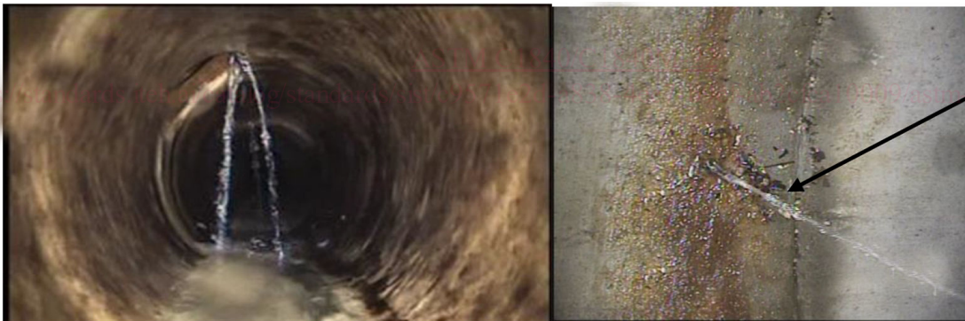
FIG. 12 Level 3 Infiltration
