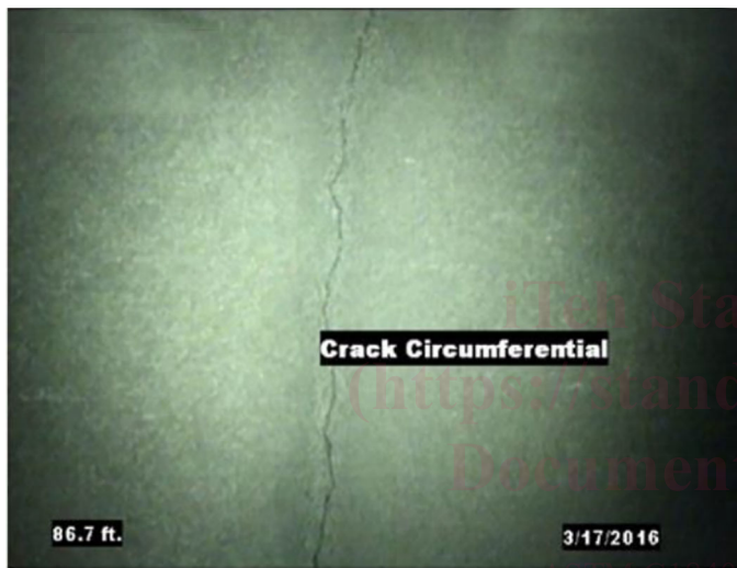
FIG. 6 Circumferential Crack
