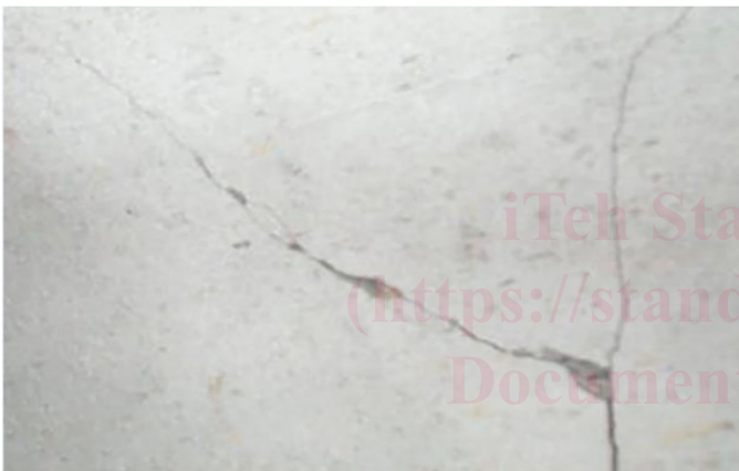
FIG. 9 Multi-Directional Crack
