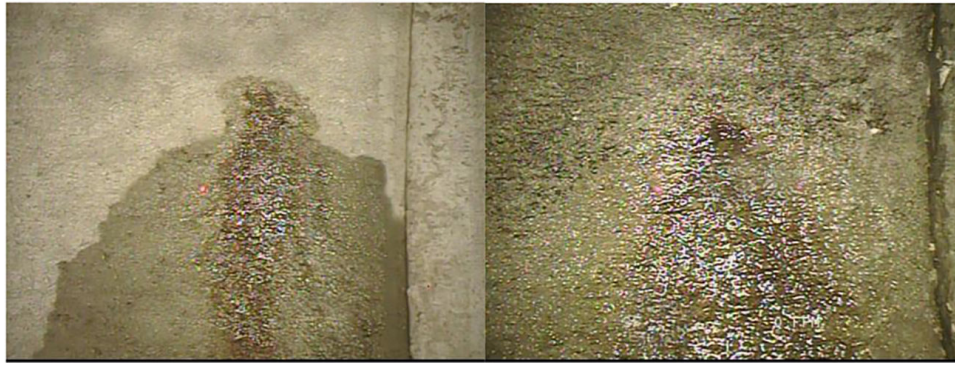
FIG. 10 Level 1 Infiltration
