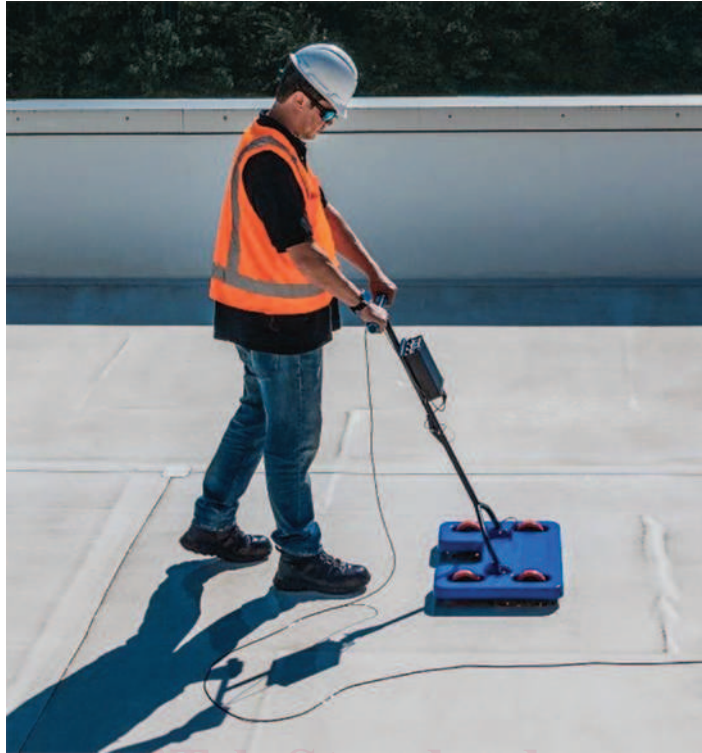
FIG. 2 Testing a Membrane with a Scanning Platform
