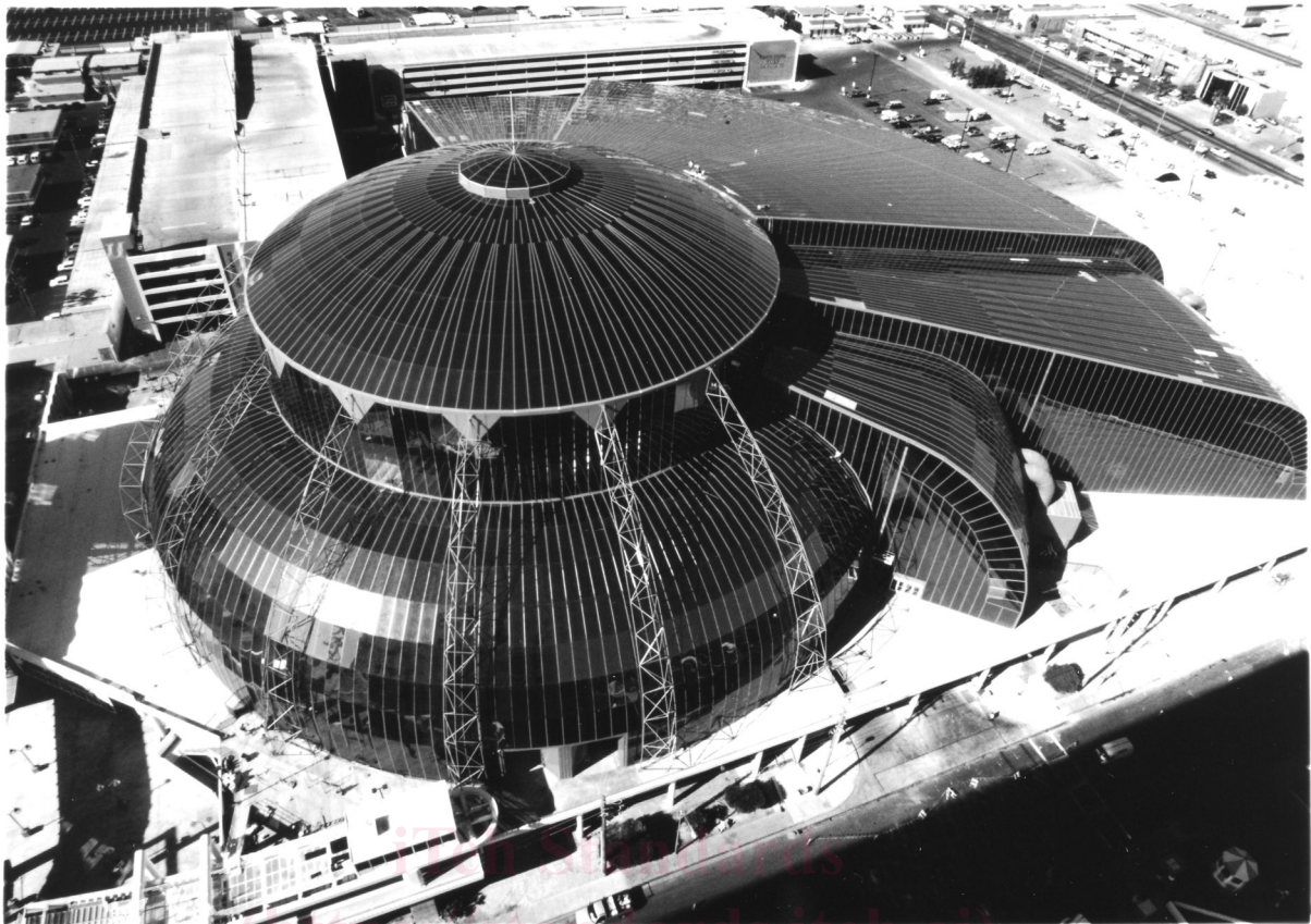
FIG. 5 Sloped SSG System
