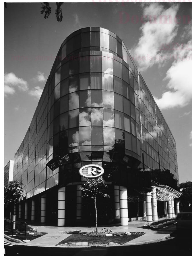
FIG. 3 Four-Side SSG System
