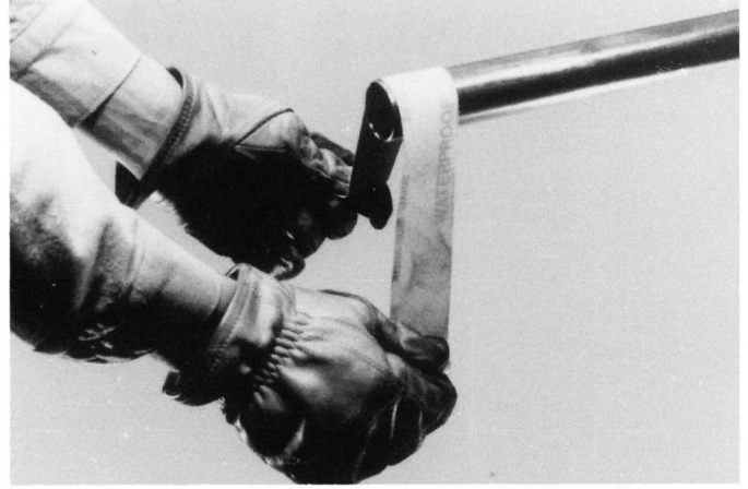
FIG. 6 Cleaning: Sand Cloth
