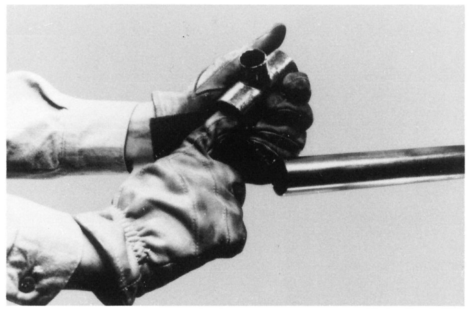
FIG. 8 Cleaning: Abrasive Pad
