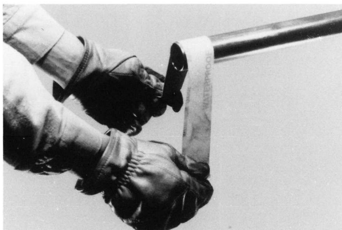
FIG. 6 Cleaning: Sand Cloth
