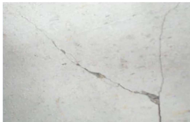
FIG. 9 Multi-Directional Crack
