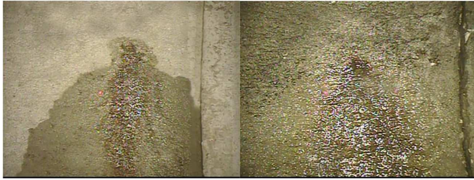
FIG. 10 Level 1 Infiltration
