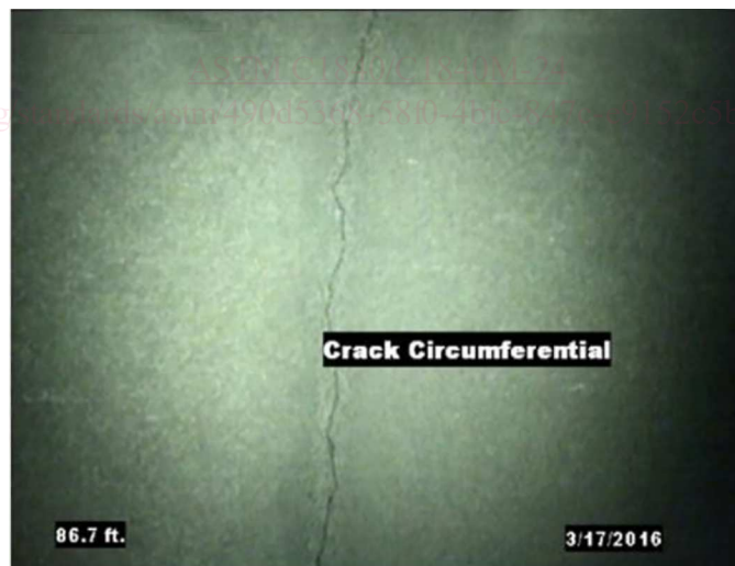
FIG. 6 Circumferential Crack
