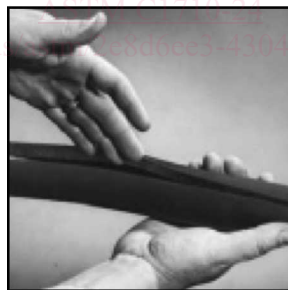
FIG. 3 Apply Unslit Insulation to Straight Pipe
