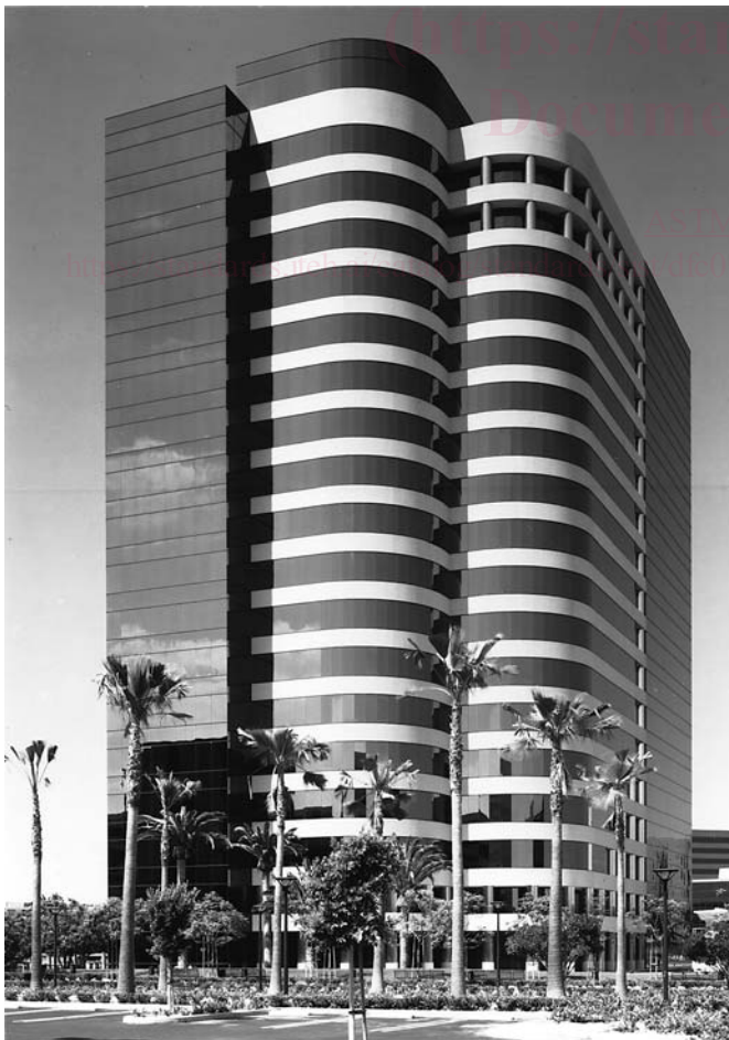
FIG. 3 Two-Side SSG System
