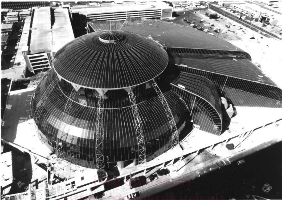
FIG. 6 Sloped SSG System
