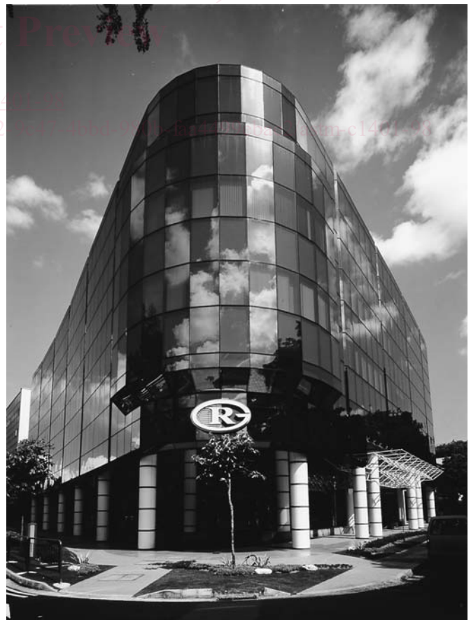
FIG. 4 Four-Side SSG System
