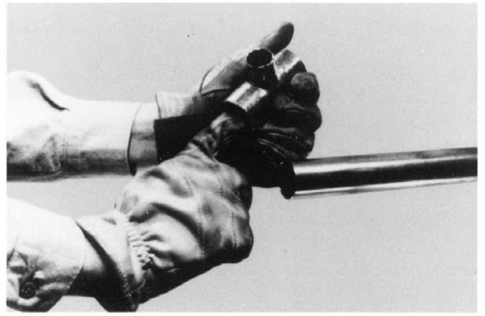
FIG. 8 Cleaning: Abrasive Pad
