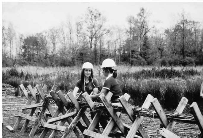
FIG. 1 Photograph of Live Fascine Fabrication (Tied Bundles, Not Installed)
