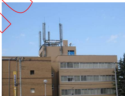
Figure 5 – Roof-top case study with large antennas and no direct access
