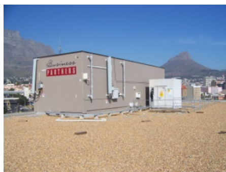
Figure 4 – Roof-top case study with direct access to antennas
