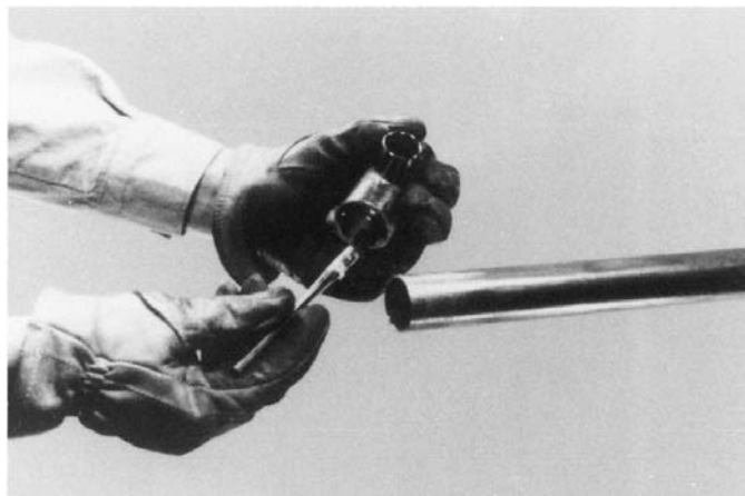
FIG. 11 Fluxing: Fitting
