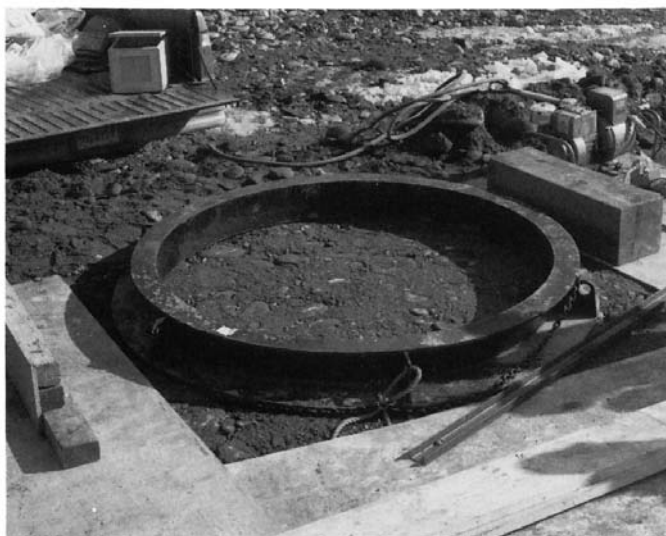
FIG. 1 A 6-ft (1.8-m) Diameter Metal Ring for Determining In-Place Unit Weight
