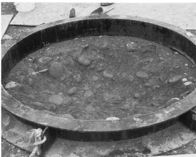
FIG. 4 Test Pit During Excavation
