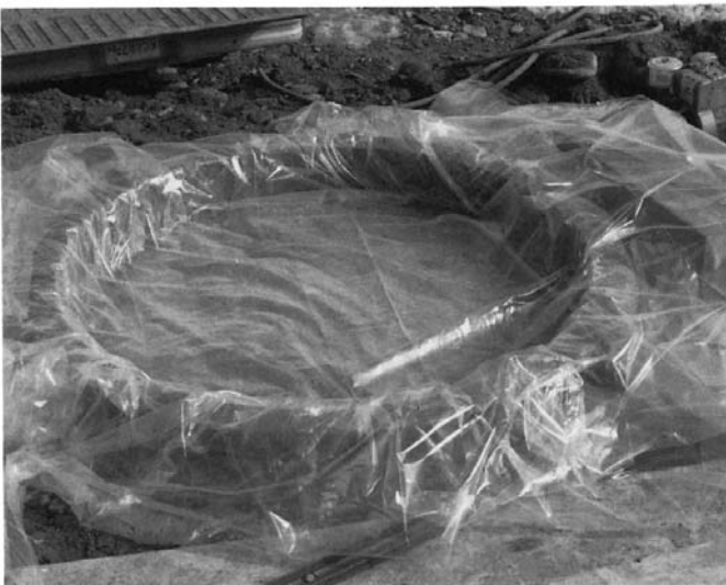
FIG. 2 Plastic Liner Placed in Preparation for the Initial Volume Determination
