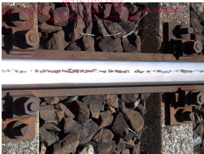
Figure 5 — Spalling
