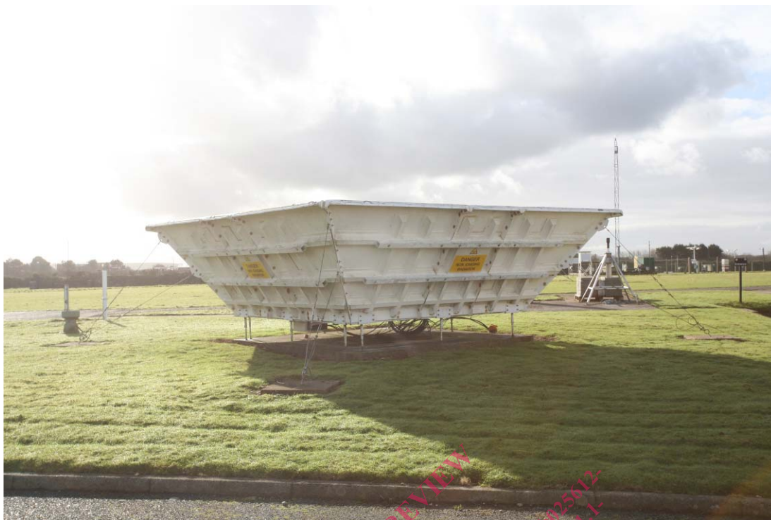
Figure 2: WPR Antenna housing
