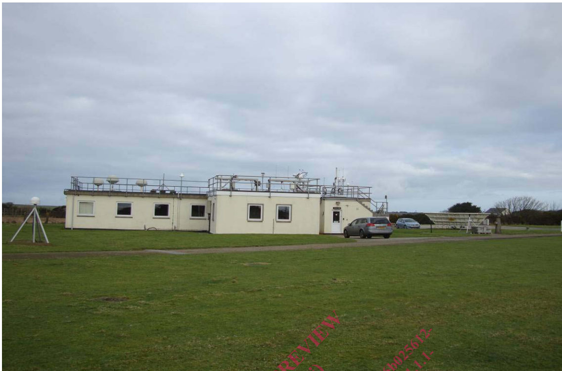
Figure 5: Tests carried out in left hand room of the building
