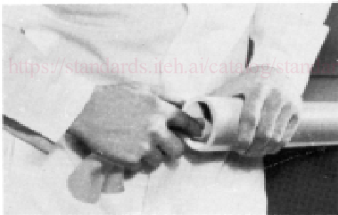
FIG. 8 Cleaning of Pipe with Dry Cloth to Remove Foreign Matter
