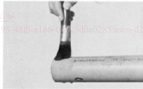
FIG. 10 Liberal Application of Primer to Soften Surface of End of Pipe
