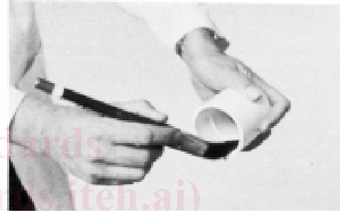
FIG. 9 Application of Primer to Inside Socket Surface
