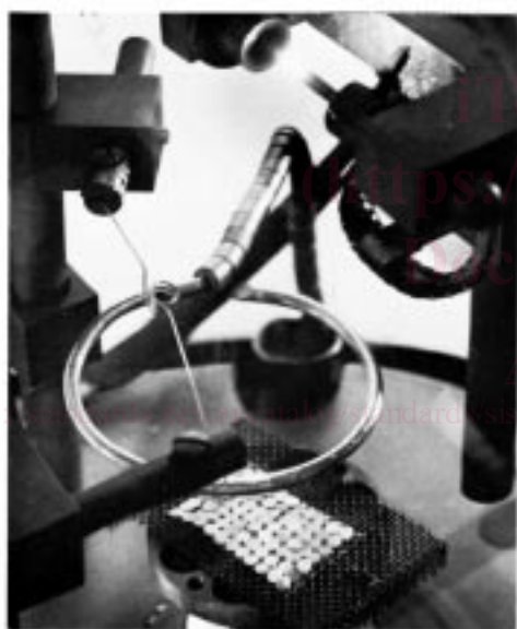
(a) Removal of Poly (Vinyl Formal) Coated Grids from the Water
