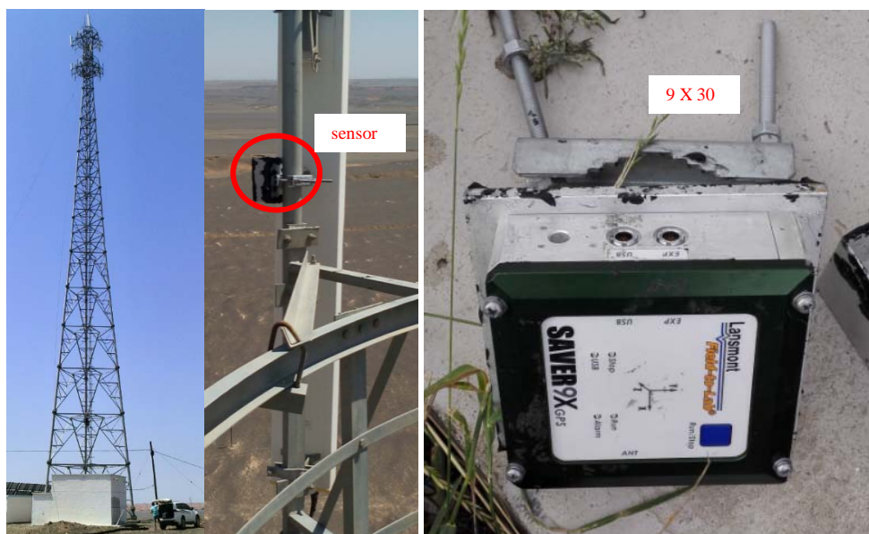
Figure 1: 60 m triangular lattice tower and mounting location
