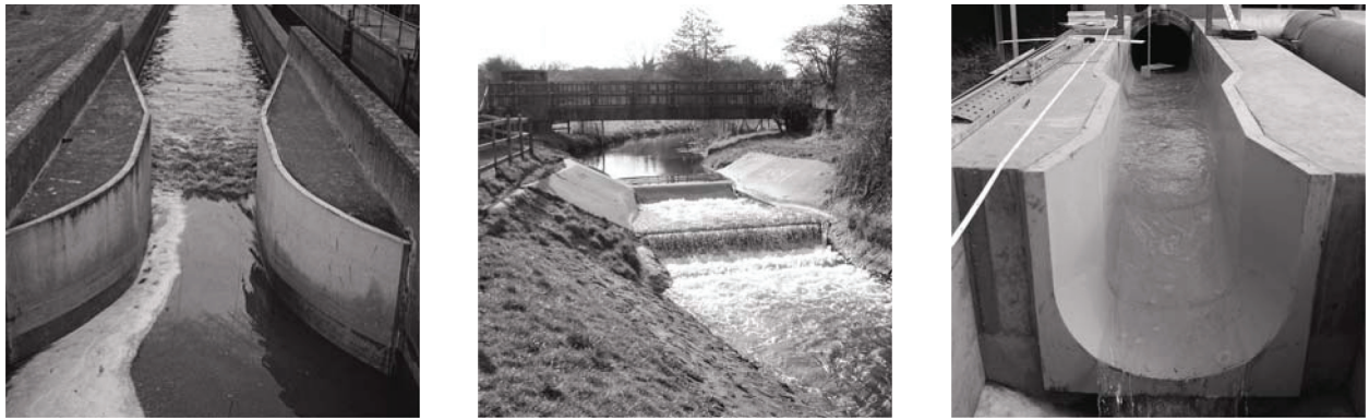
a) Rectangular-throated flume b) Trapezoidal-throated flume c) U-throated flume
