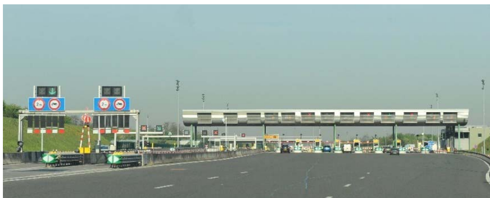
Figure 2: Toll plaza with non-stop ETC lanes (left), stop&go ETC and automatic lanes (right)
