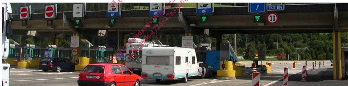
Figure 1: Toll plaza with non-stop ETC lane (far left), stop&go ETC (centre lanes) and automatic lane (right)
