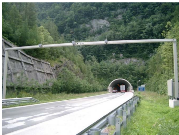
Figure 4: Typical free-flow installation with three lanes
