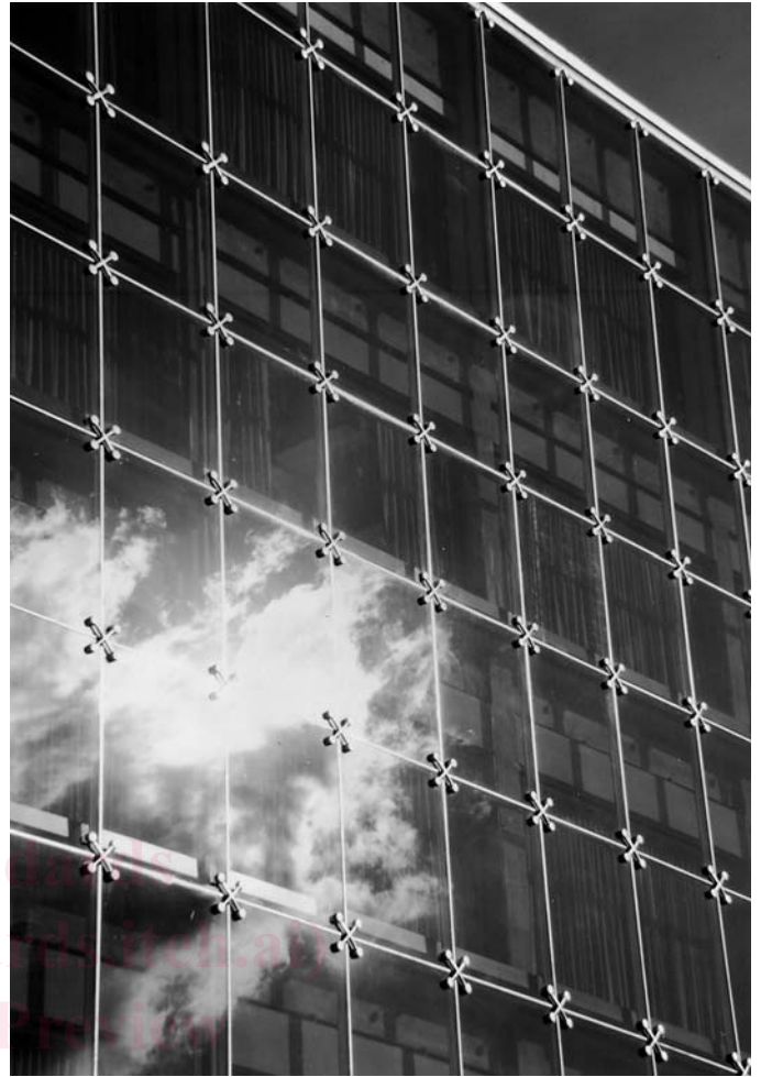
FIG. 4 Four-Side SSG System
