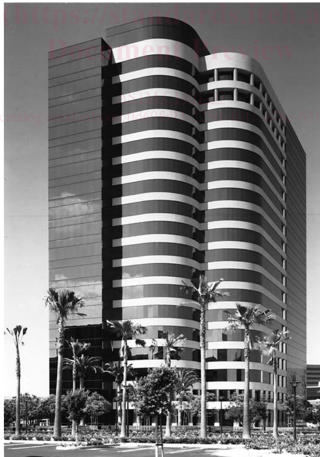
FIG. 2 Two-Side SSG System
