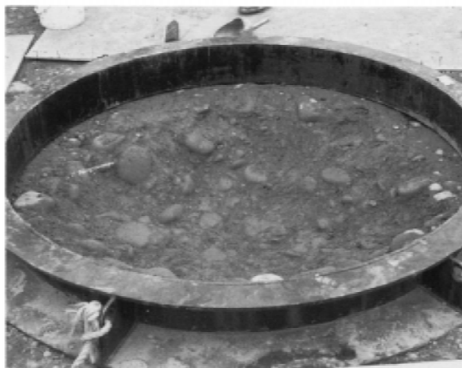
FIG. 4 Test Pit During Excavation
