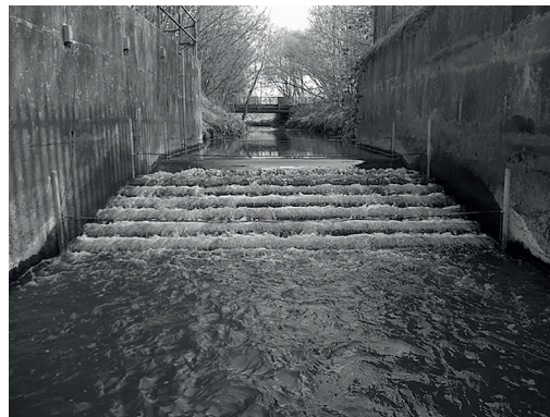
b) Flow condition on a weir with baffles under running condition
