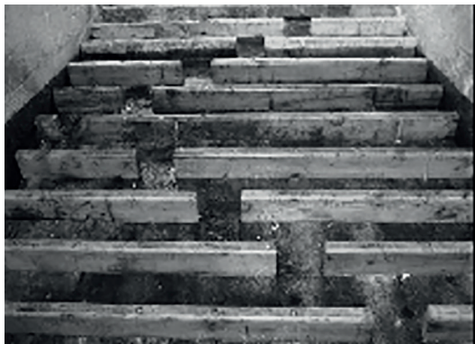
a) Baffles installed on a weir shown under dry conditions
