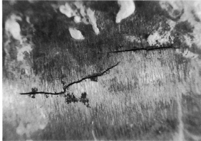
FIG. 2 Typical External Stress Corrosion Cracks (5× Magnification)
