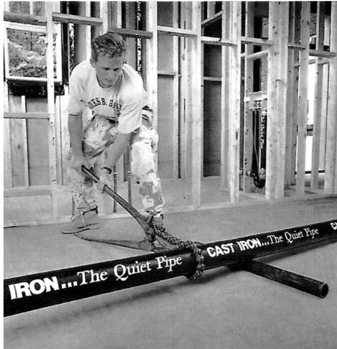
FIG. X1.1 Snap Cutter
