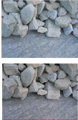
Figure 1 — Drainage aggregate in contact with protection geotextile
