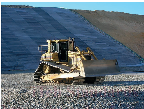
Figure 2 — Placement of drainage aggregate
