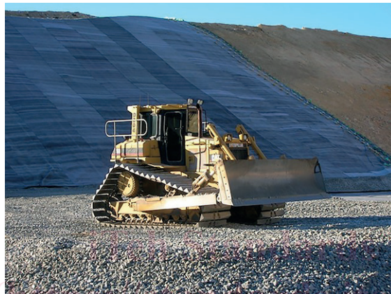
Figure 2 — Placement of drainage aggregate
