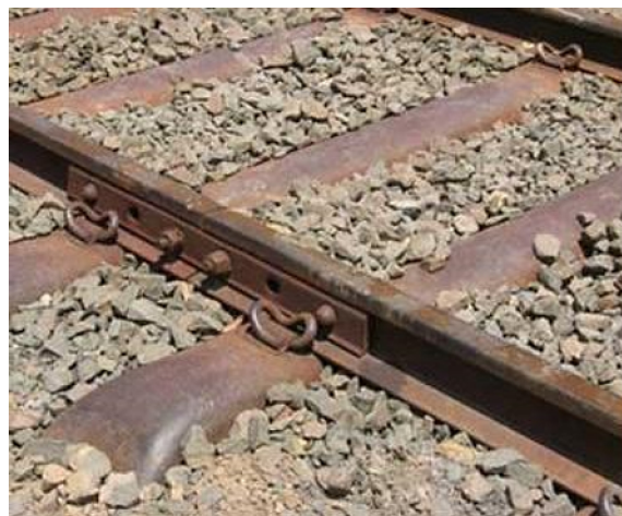
b) Steel sleepers
