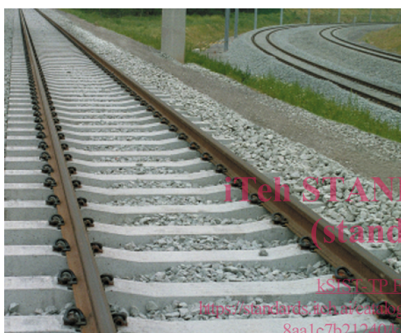
c) Mono-block sleepers
