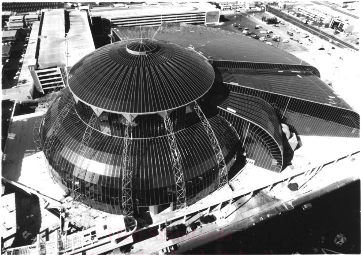
FIG. 5 Sloped SSG System
