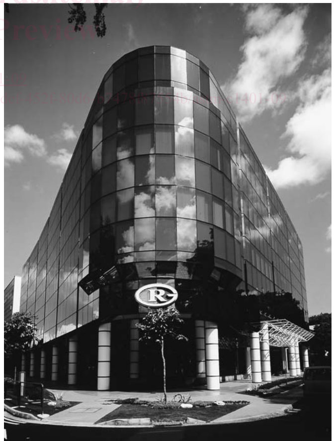
FIG. 3 Four-Side SSG System
