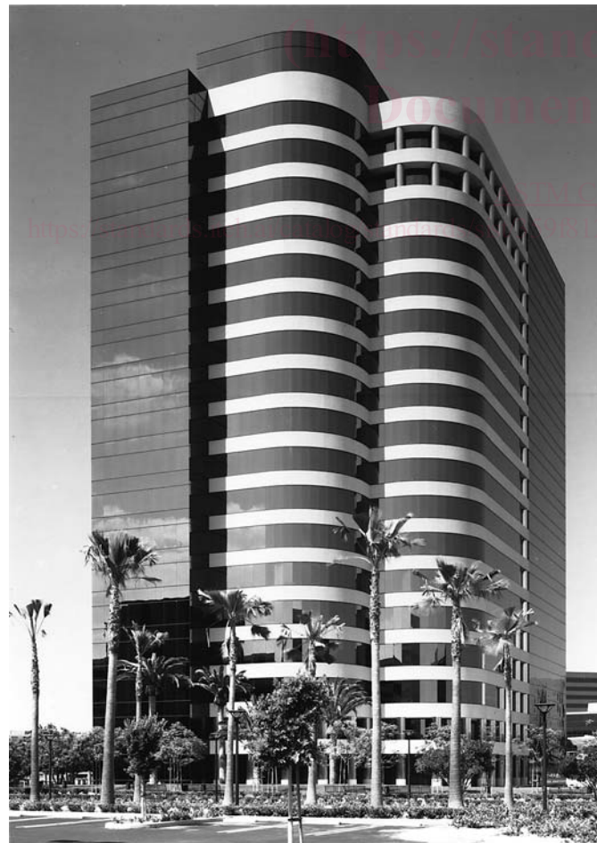
FIG. 2 Two-Side SSG System
