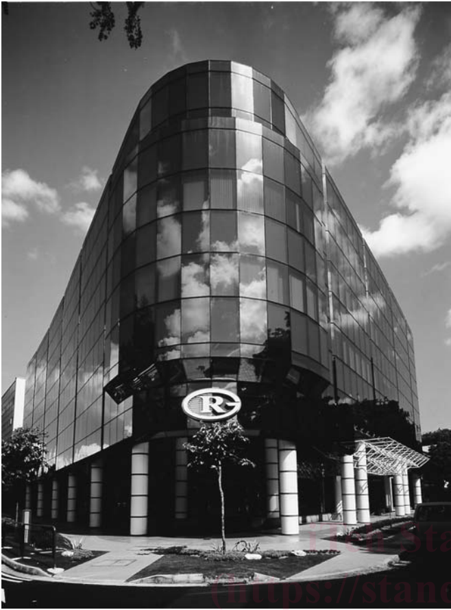
FIG. 3 Four-Side SSG System
