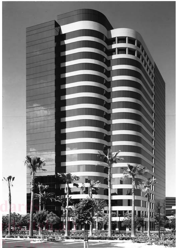
FIG. 2 Two-Side SSG System
