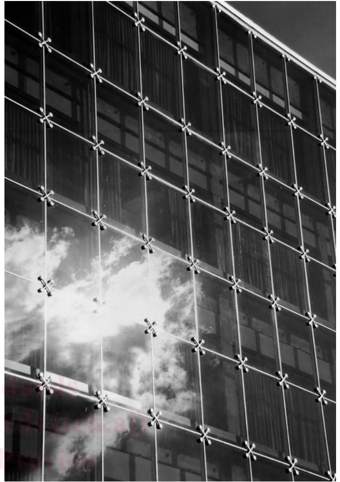
FIG. 4 Four-Side SSG System
