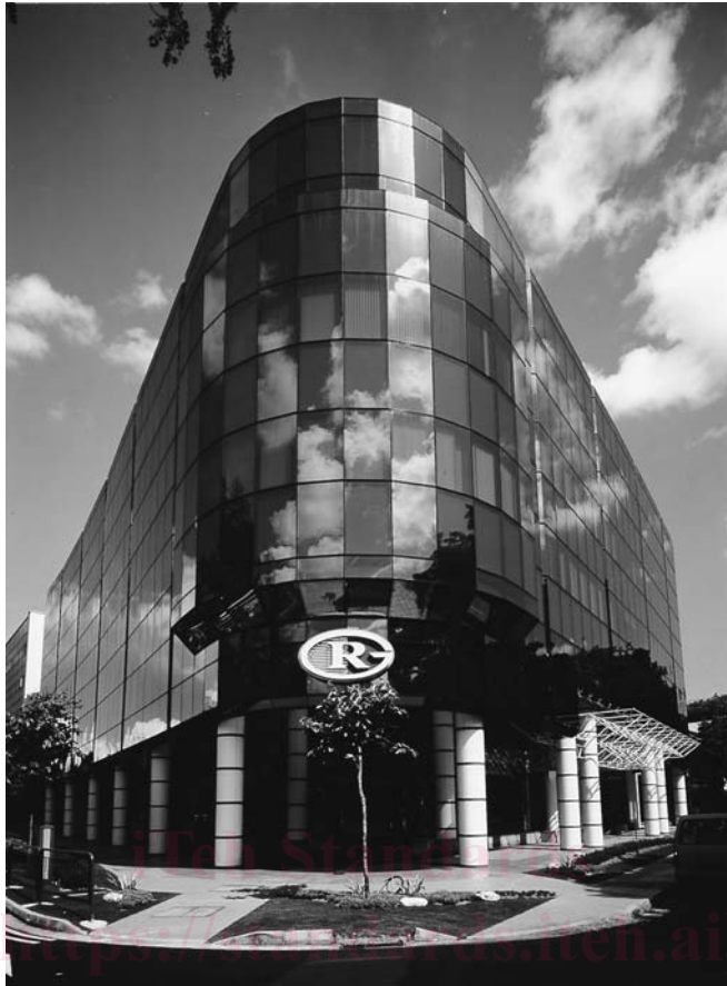
FIG. 3 Four-Side SSG System
