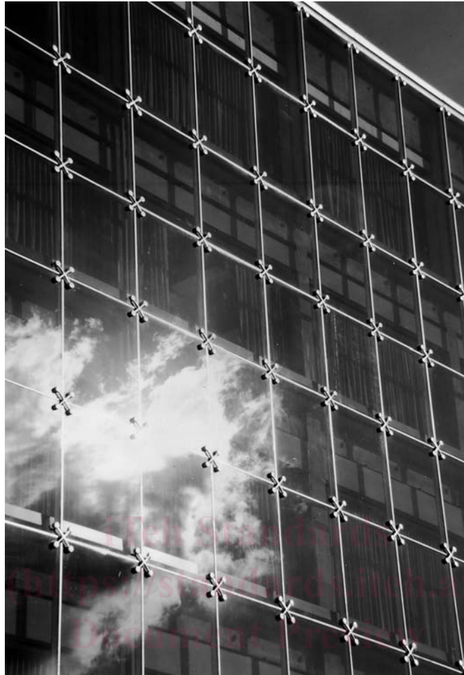
FIG. 4 Four-Side SSG System
